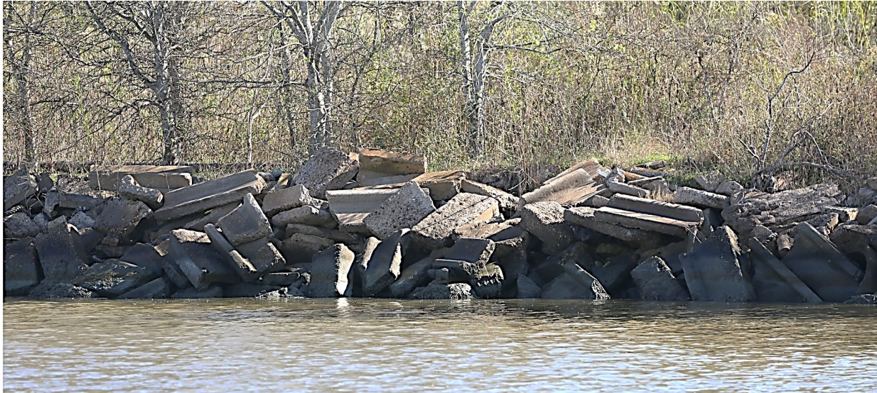
Figure 1-3. Typical Non-Engineered Shoreline of Pleasure Island
